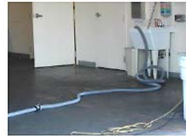
Discharge to utility sink
